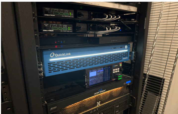
Quicklink scene-based production switcher—the central control system powering Westminster’s flexible broadcast studio.
